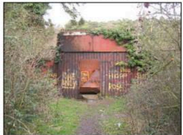
"Security" sheeting to south end of bridge
