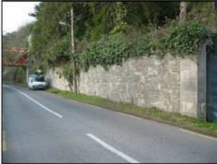
Retaining wall to north abutment approach
