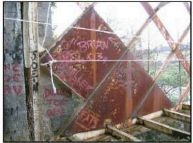
Later steel security sheeting welded to girders
