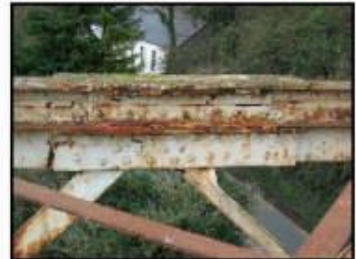
Splice detail top boom
