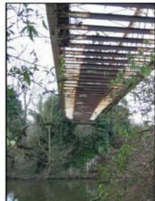
South Abutment viewed from north bank
