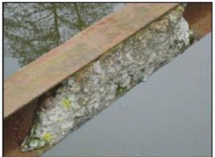
Detail of clinker concrete between deck beams
