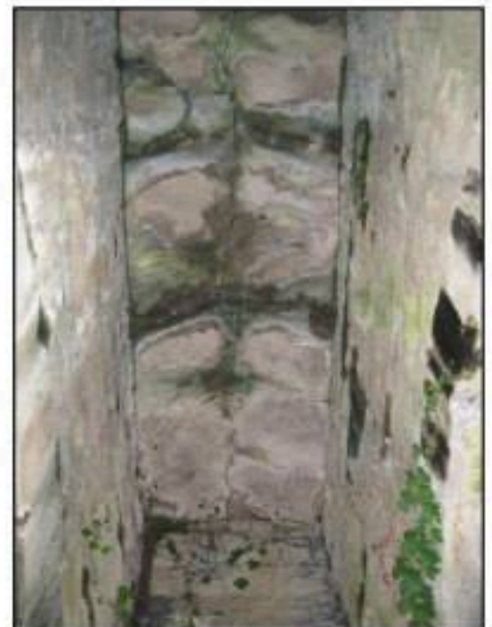
North abutment u/s roof, note rwdp in corner
