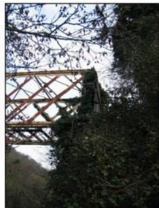
South Abutment, note ivy
