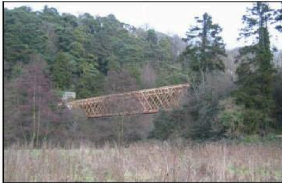
View of bridge from south bank looking northeast
