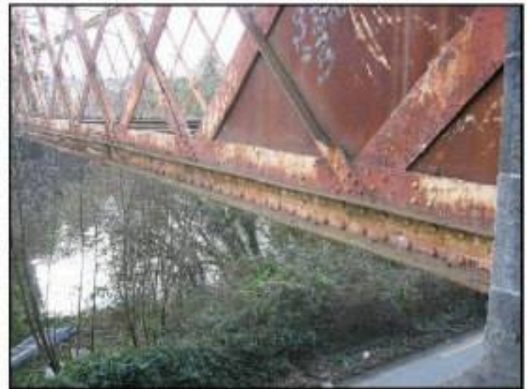
South girder bottom boom at north abutment
