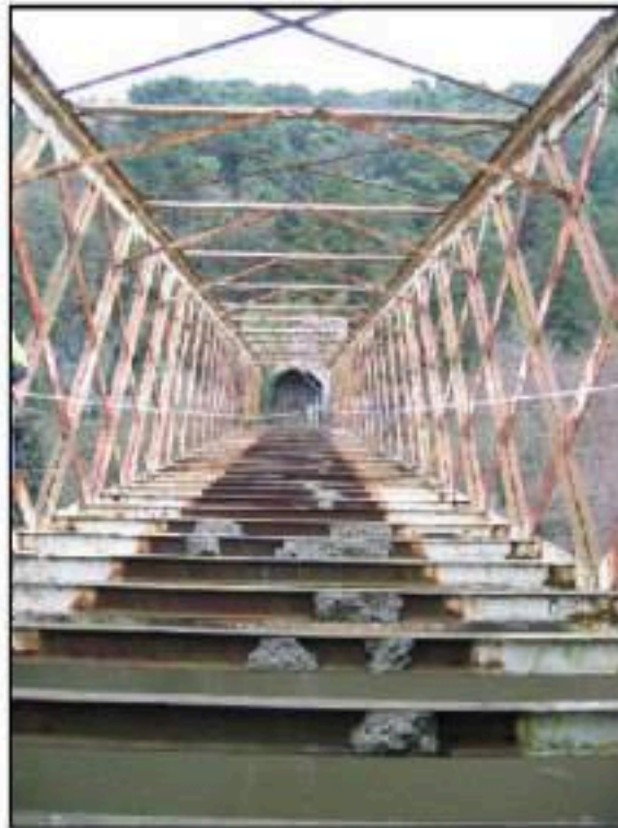
View on deck looking north
