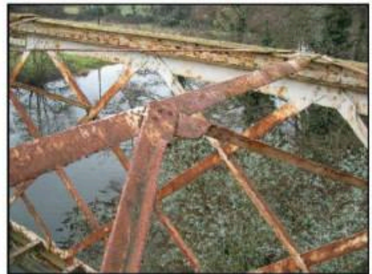
Bracing detail between top of girders
