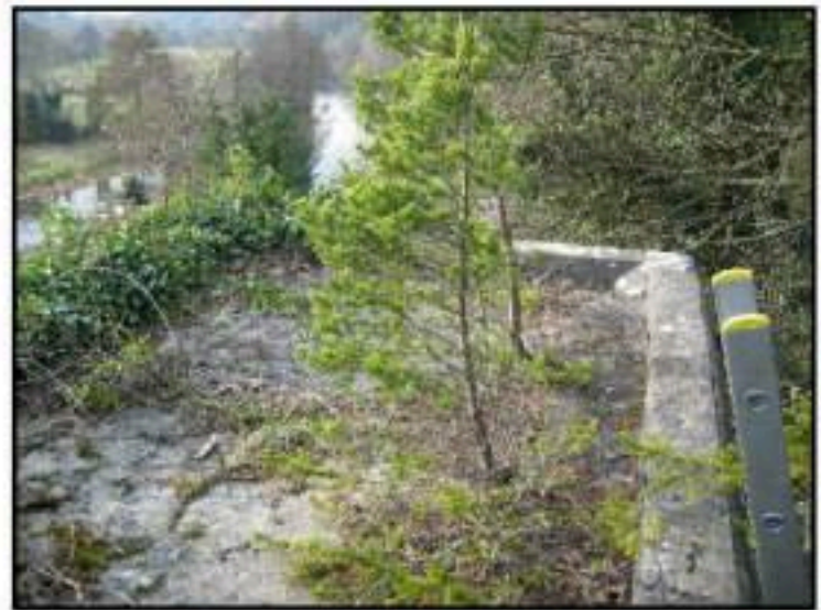
North abutment – roof garden
