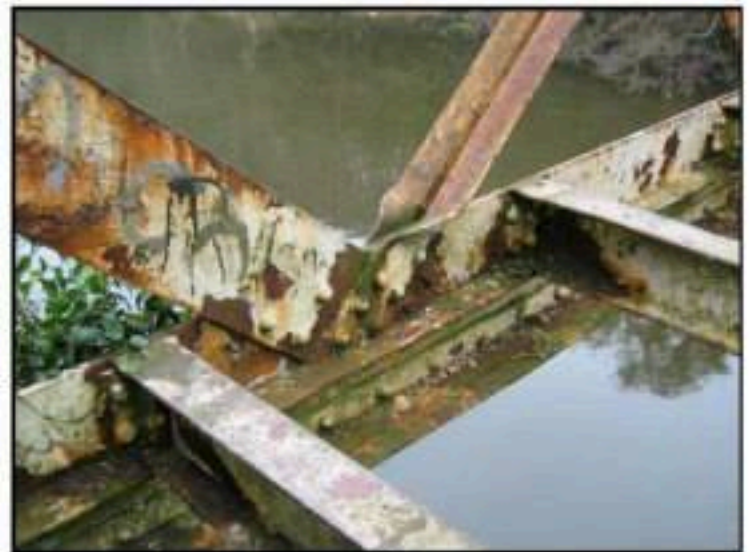
Detail of bottom boom and deck beam connection
